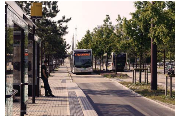
Figure 9.3 Nantes guided busway
