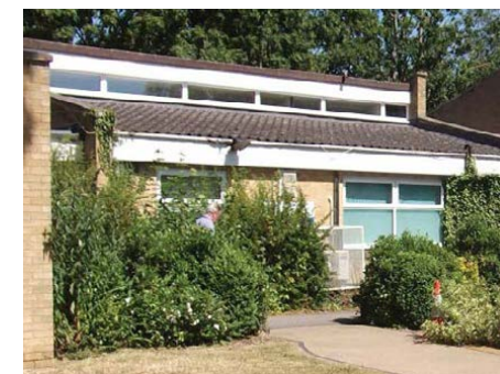
Figure 4.7 Health centre, Exeter Close
