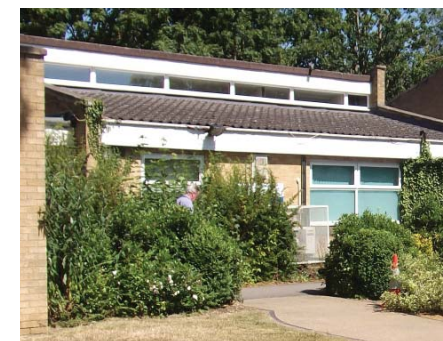
Figure 2.16 Health centre, Exeter Close
