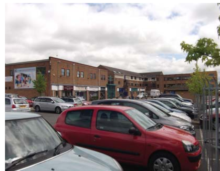
Figure 2.14 Surface car parking
