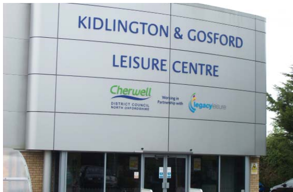
Figure 2.20 Gosford - leisure centre
