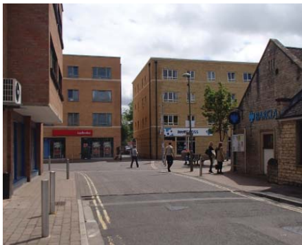
Figure 4.17 Poor quality design of prominent recent schemes
